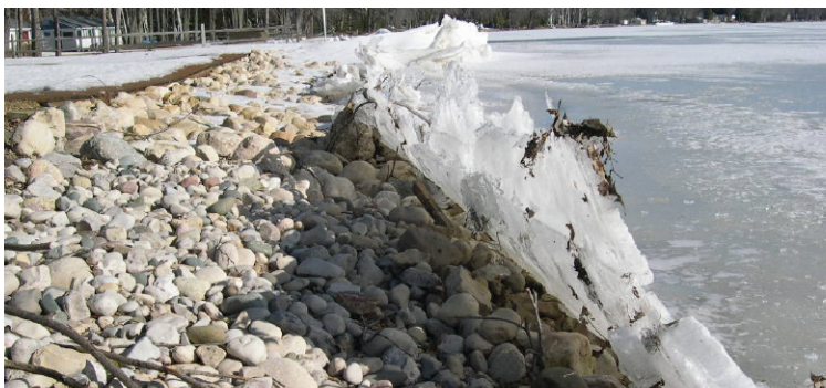
This higher-energy bioengineering project is protecting this shoreline from ice-push. Photo courtesy of Jennifer Buchanan, Tip of the Mitt Watershed Council.
