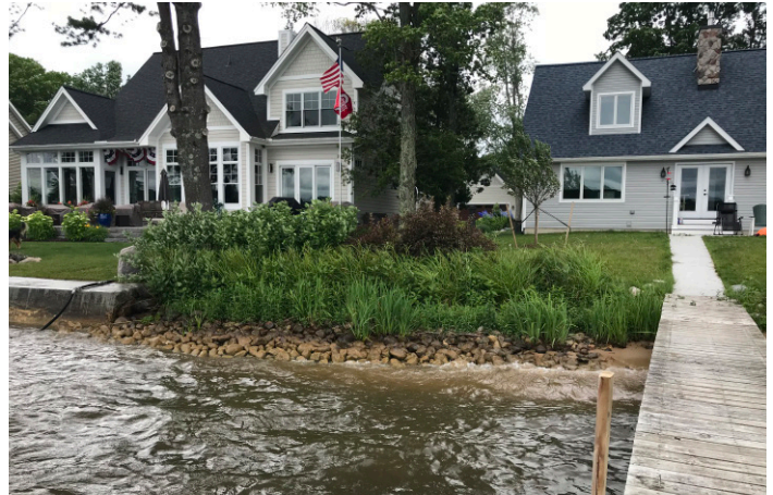
This bioengineering design protects the shoreline on this high energy lake by dissipating wave energy from wind and boats while still providing lake access and not impeding lake views. Photo courtesy of Jennifer Buchanan, Tip of the Mitt Watershed Council.
