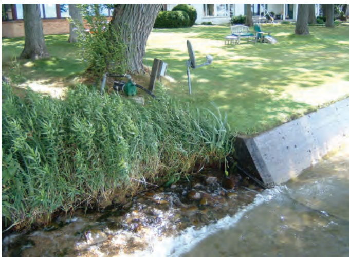
Figure 4.20. No-mow zone unable to withstand waves projected from the neighboring seawall (July 2007). (Photo: Jane Herbert.)
