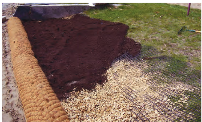
Figure 4.29. Gravel and topsoil fill reinforced with vinyl geoweb. (Photo: landowner.)
