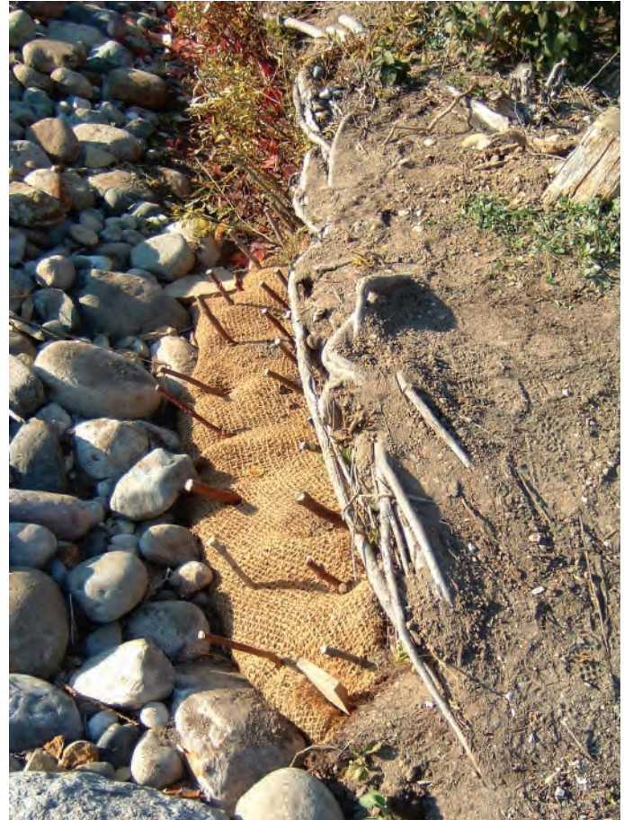
Figure 4.16. Autumn installation of dormant live stakes (foreground) and whips to repair shoreline damaged by an uprooted tree. (Photo: Jane Herbert.)
