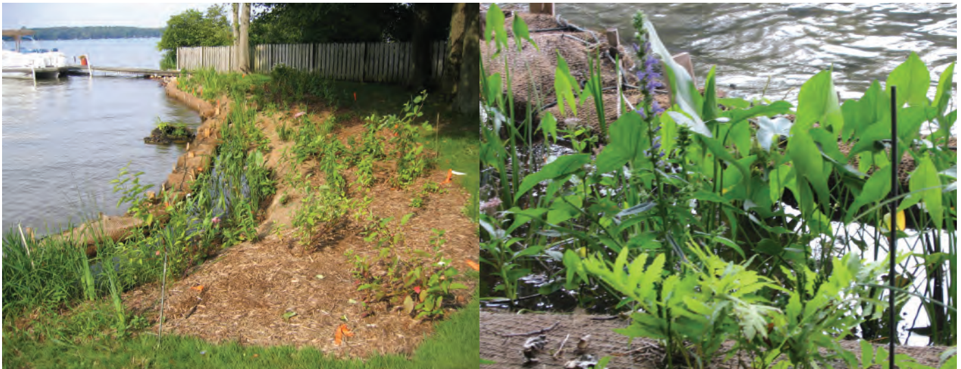
Figure 4.11. Bioengineered erosion control and buffer strip of native wetland and aquatic plants at seven weeks after installation. Gull Lake, Kalamazoo County, Mich. (Photos: Jane Herbert.)
