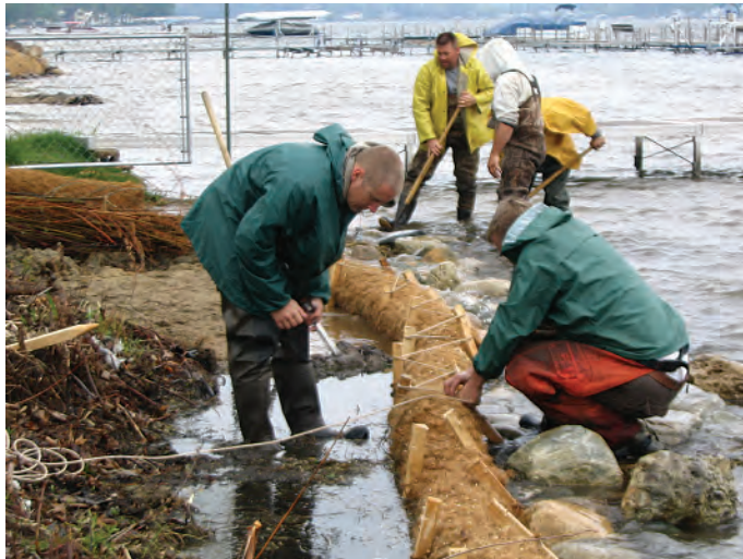
Figure 4.25. Lashing down staked coir logs with nylon rope (foreground). Previously placed stones are being rearranged by hand. (Photo: JFNew.)
