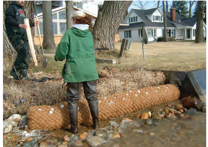
Figure 4.21. Coir log installation, March 2008. (Photo: Jane Herbert)
