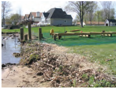
Figure 4.24. Eroding shoreline before the installation of a native plant buffer strip (spring 2005). (Photo: JFNew.)
