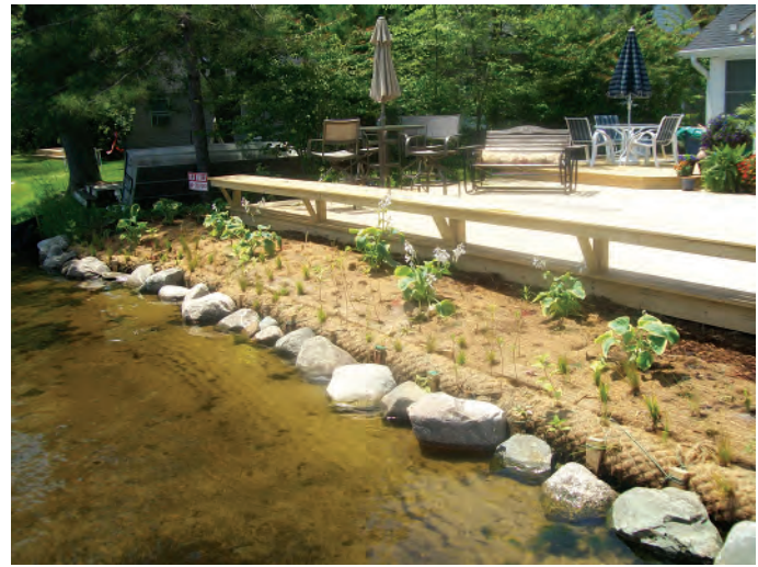
Figures 4.19. “After” picture. Erosion control included a mix of soft- and hard-arming techniques to stabilize the shoreline and offer protection from erosive forces. (Photo: Jane Herbert.)
